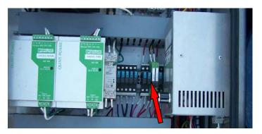
This breaker MUST be opened to prevent damage to the winch valve manual actuator linkage.
